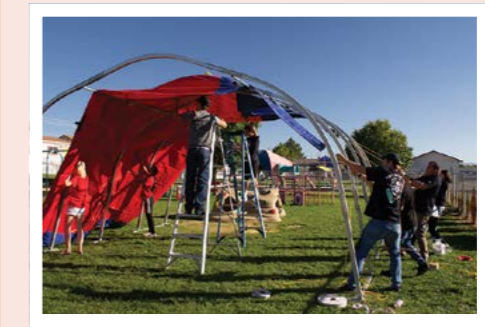
Volunteers assemble the outdoor shade structure at a local elementary school.
